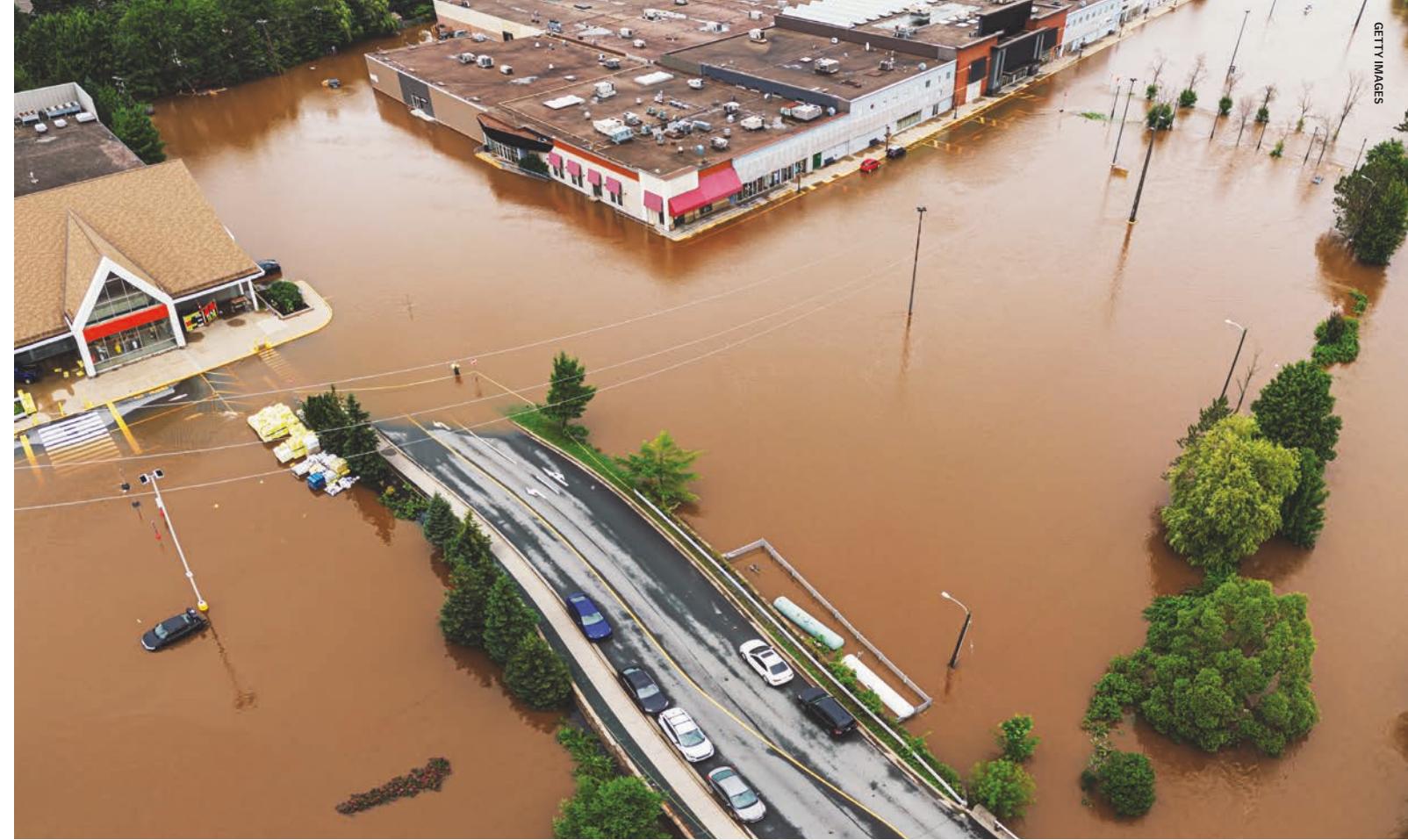
Clients should store their critical machinery, equipment, inventory stock, spare parts and importantly, IT servers, in locations that have been thoroughly assessed and reviewed for potential risks.
